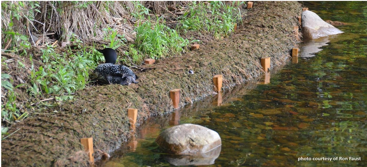
Shoreline restoration using coconut fiber-based coir logs, restoring habitat for clean water
